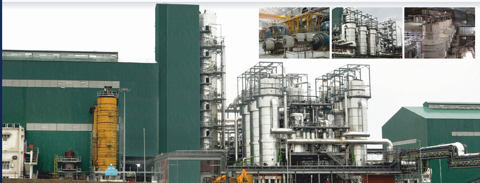
10000 TCD Refined Sugar Plant with 210 TPH / 125 Bar, Bagasse Fired Boiler and 40.5 MW Power Plant, having all FFE & VCP designed on 30% Steam on cane at KPR Sugars, Karnataka, India
