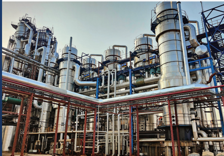
10000 TCD Refined Sugar Plant with 210 TPH / 125 Bar, Bagasse Fired Boiler and 40.5 MW Power Plant, having all FFE & VCP designed on 30% Steam on cane at KPR Sugars, Karnataka, India
