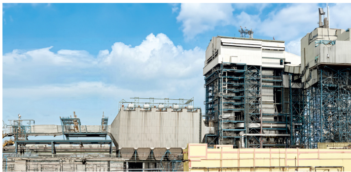
Reheat type Cogeneration Multi Fuel Fired Circulating Fluidised Bed Combustion (CFBC) Boiler, designed for six different operating conditions of process steam and turbine.
