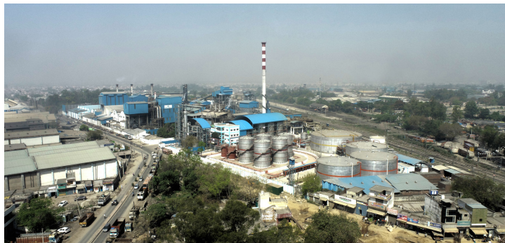
160 KLPD multi-feed Ethanol Plant with 48 TPH Slop Fired Incineration Boiler and 5.6 MW Power Plant.
