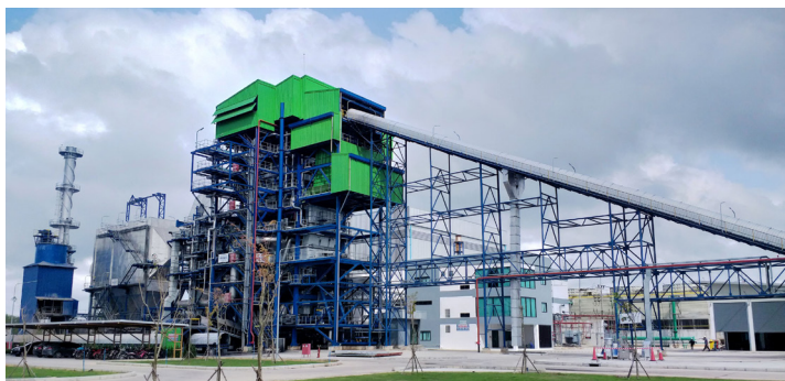
Reciprocating Grate Boiler for burning empty fruit bunch (bulky fuel with high alkali, chlorine, and oil content) for a plant in Thailand.
