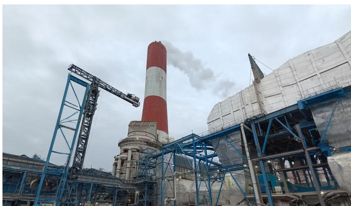
First to commission the largest Wet FGD in India for an 800 MW thermal power unit which will reduce more than 96% of the SO 2 emissions generated by the unit, thereby producing saleable gypsum as by-product.
