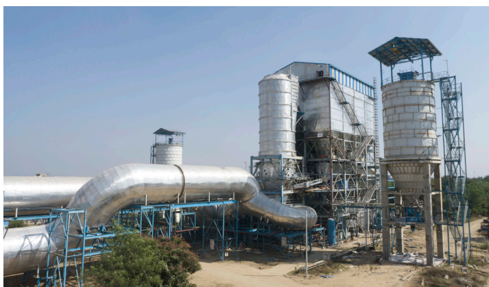
First Semi Dry FGD based on Circulating Fluidised Bed Scrubber Technology commissioned in India for a 150 MW thermal power unit.
