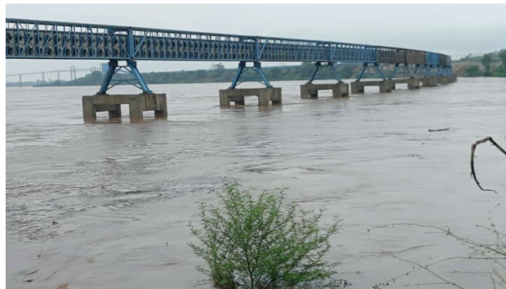
16 km Pipe and Trough Conveyor System for transportation of coal from three mines to two thermal power plants crossing two rivers and several railway lines, in Western India.
