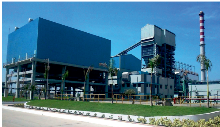
30 MW Captive Power Plant with Circulating Fluidised Bed Combustion Boiler on turnkey basis.
