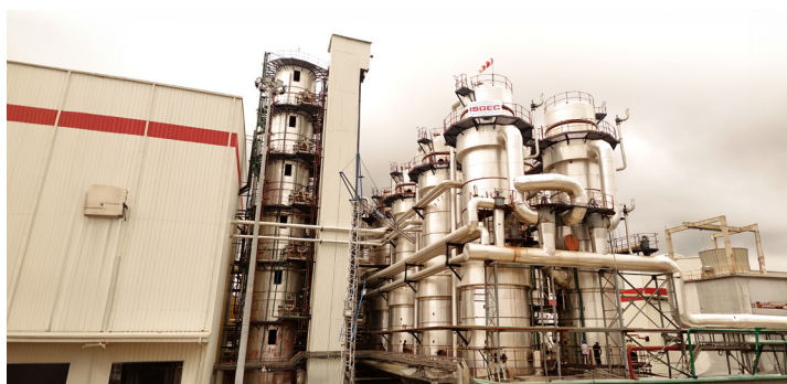
7,500 TCD integrated Sugar Complex in North India with 26% process steam consumption on cane.
