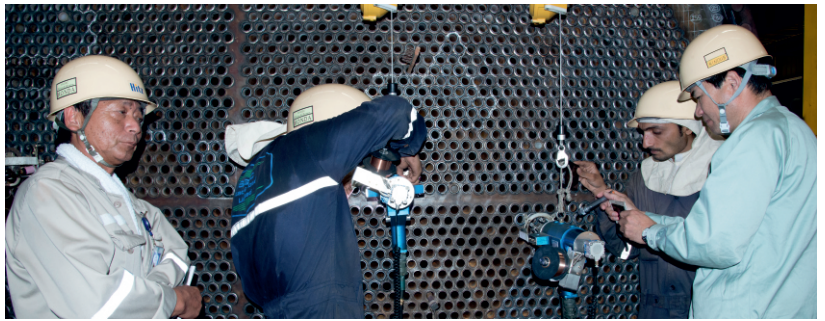
Automatic Tube to Tube Sheet Welding in EO Reactor
