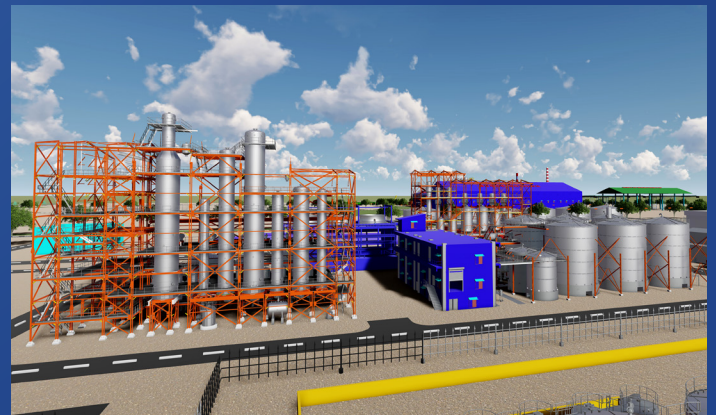
3D Plant View: 210 KLPD ENA Plant with 32 TPH Slop Fired Boiler, West Kenya Sugar Company, Kenya, India
