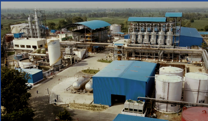
175 KLPD Distillery Plant with 44 TPH Slop Fired Boiler & 5 MW Power Plant (Repeat Order), Dwarikesh Sugar Industries Ltd., Bareilly, India
