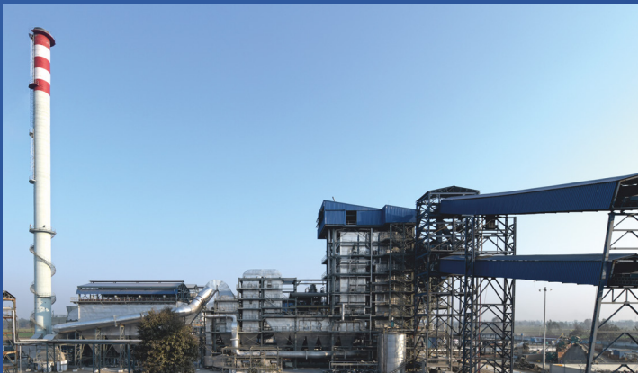
80 TPH, 45 kg/sq.cm. (g), 400 Deg. C, Slop / Bagasse Fired Travelling Grate Boiler at DCM Shriram Sugars, Ajbapur U.P, India
