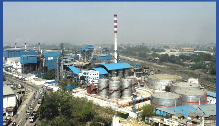
160 KLPD Distillery Plant with 48 TPH Slop Fired Boiler & 5.5 MW Power Plant including Civil Work, Saraswati Sugar Mills, Haryana, India
