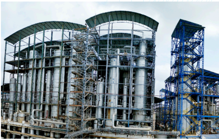
200 KLPD Distillery Plant on Syrup / B Molasses with 60 TPH Slop Fired Boiler, Mellbro Sugar Pvt. Ltd., Bagalkot, India
