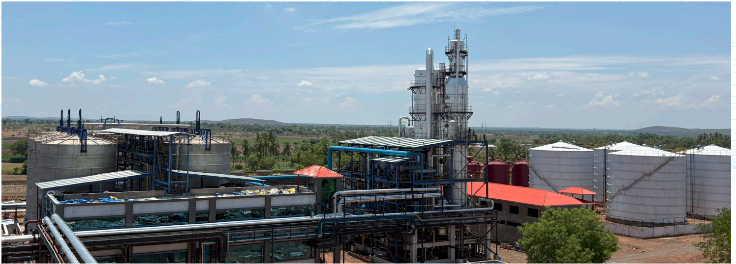
300 KLPD Multi-Feed Syrup/Molasses/Grain Distillery Plant at Kedarnath Sugar Ltd., Karnataka, India (Nirani Group - Distillation section design on 1.2 kg/cm 2 steam pressure)
