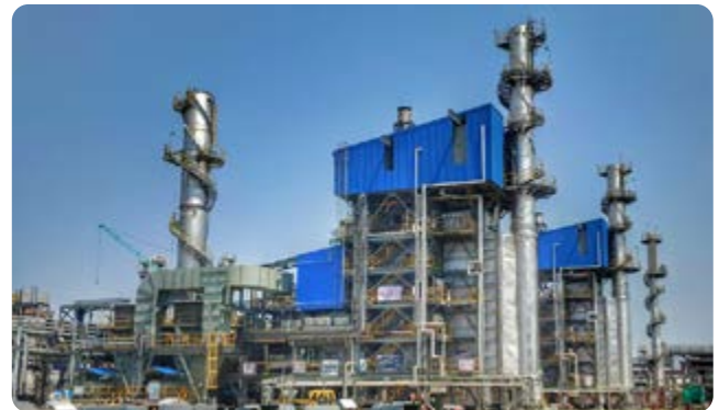
Heat Recovery Steam Generator
