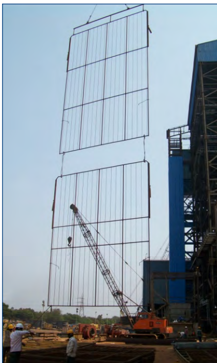
Discharge Frame with VARIODYN 15 Electrodes
